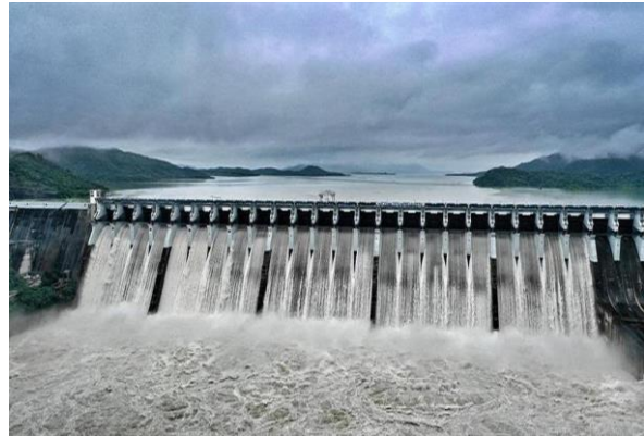
Fig. 15.1 Sardar Sarovar Dam
